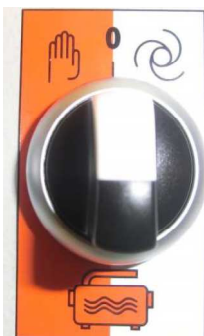
Fig. 13: Operating modes water pump
